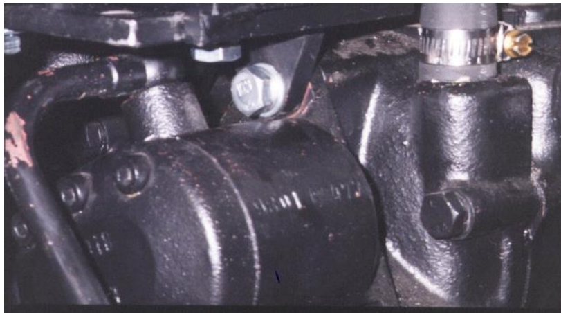
Front bolt on compressor mount.
